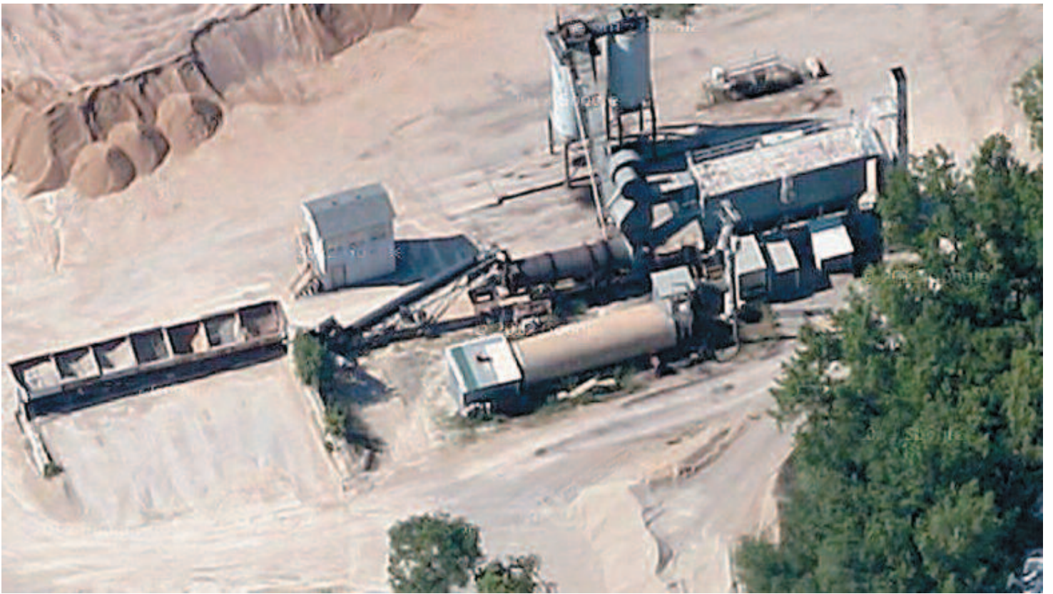
Asphalt Plant located at 936 Appleton Road • Menasha, WI 54952
